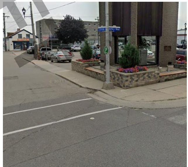
Figure 12: Traffic signal pole obstructing sidewalk in southwest quadrant of King and Centre
