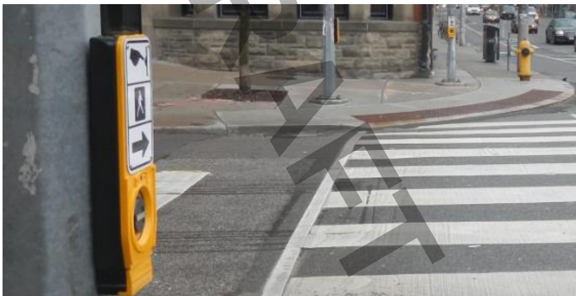
Figure 8: Accessible Pedestrian Signal (APS) front left, and Tactile Walking Surface Indicators (TWSI) along a depressed curb rear right
