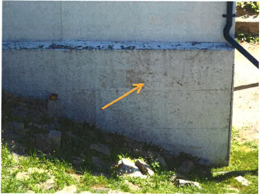
11 View of concrete foundation wall strengthening measures carried out in 1977
