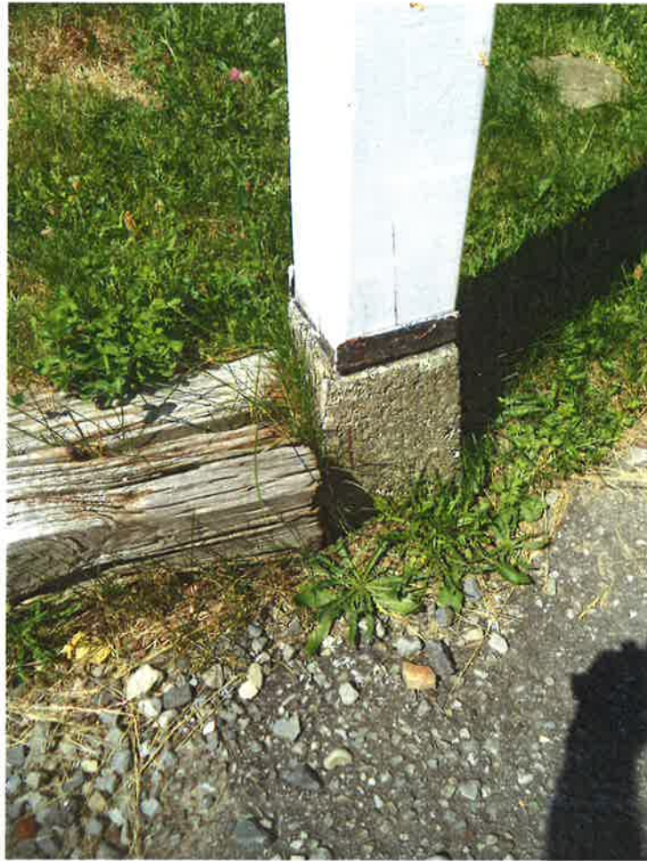
15 Typical balcony post support detail
