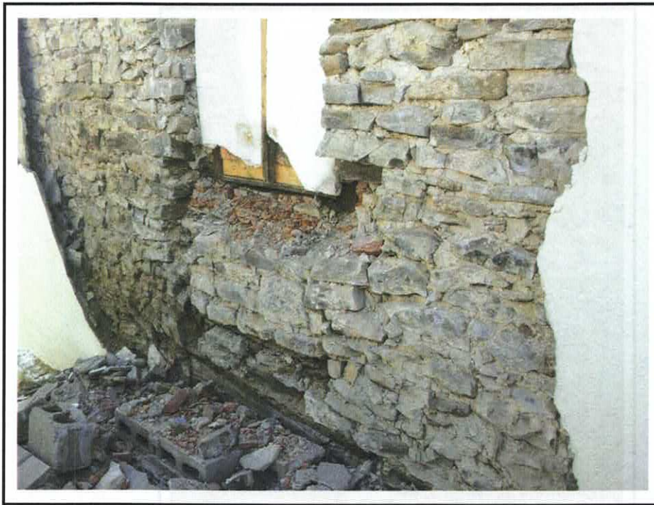
Photo 9 Deterioration at Window in East Wall
