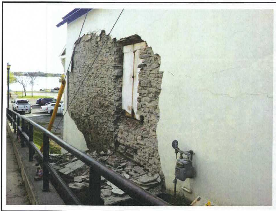
Photo 7 Removal of Stucco/Parging on East Wall
