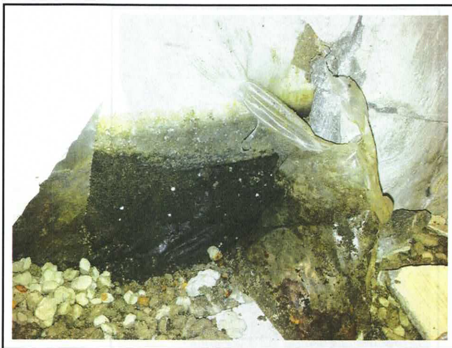
Photo 13 Insulation and Vapor Barrier where Finishes Removed in Basement (Note: staining and dampness)
