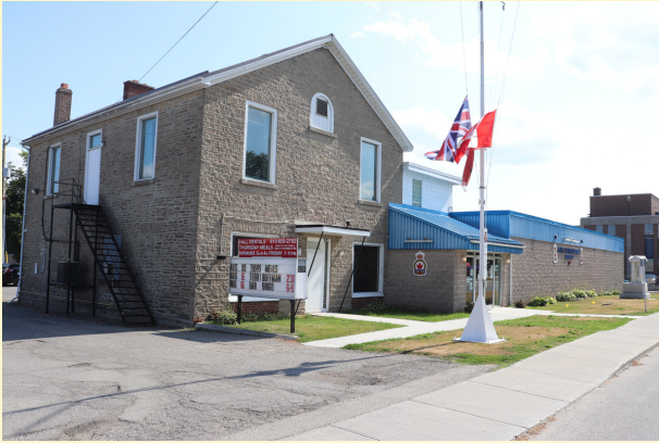
Prescott Legion Branch 97 at 141 Henry Street West
