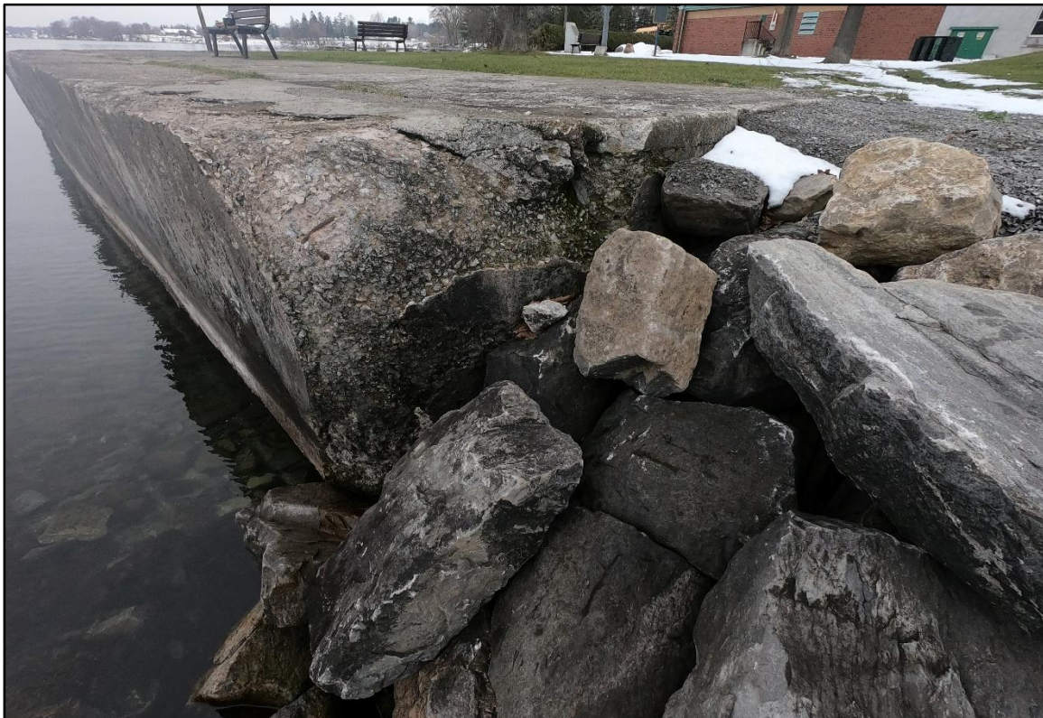
Photo 8: Existing concrete parapet at armour stone transition, SE shoreline
