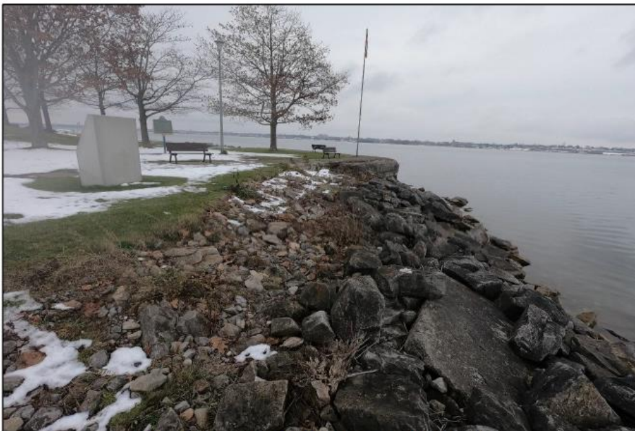
Photo 4: Existing armour stone on SW shoreline
