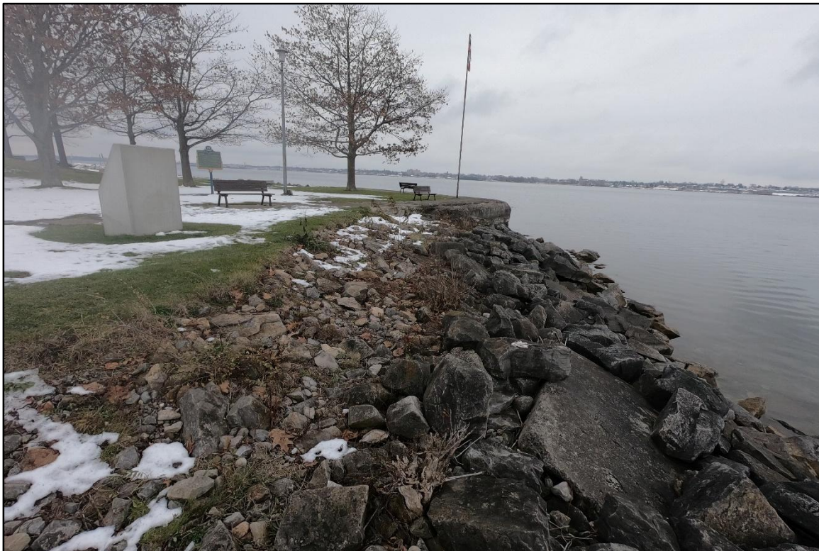
Photo 4: Existing armour stone on SW shoreline
