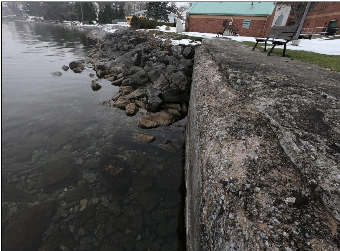
Photo 6: Existing concrete parapet, top edge of SW face
