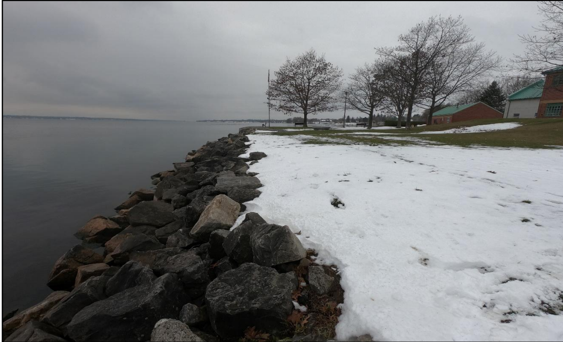
Photo 5: Existing armour stone on SE shoreline
