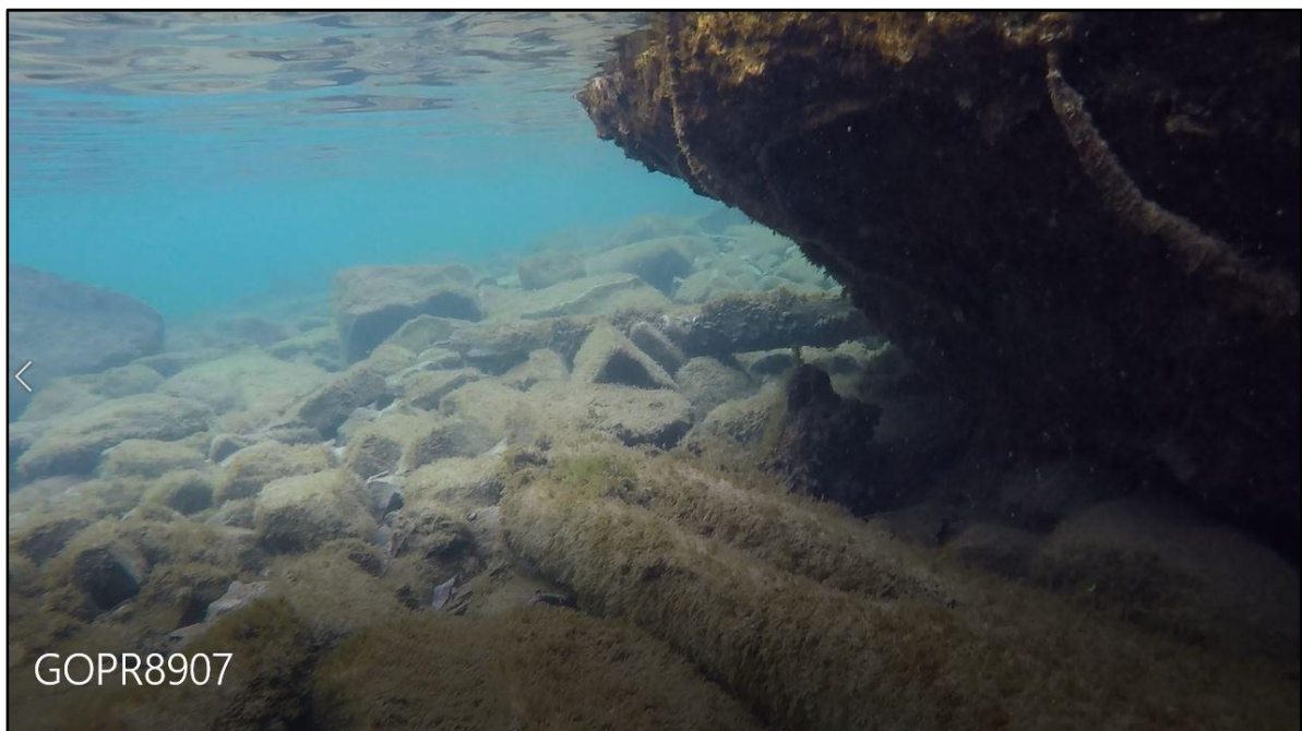
Photo 16: Failed cribbing of concrete parapet foundation at corner
