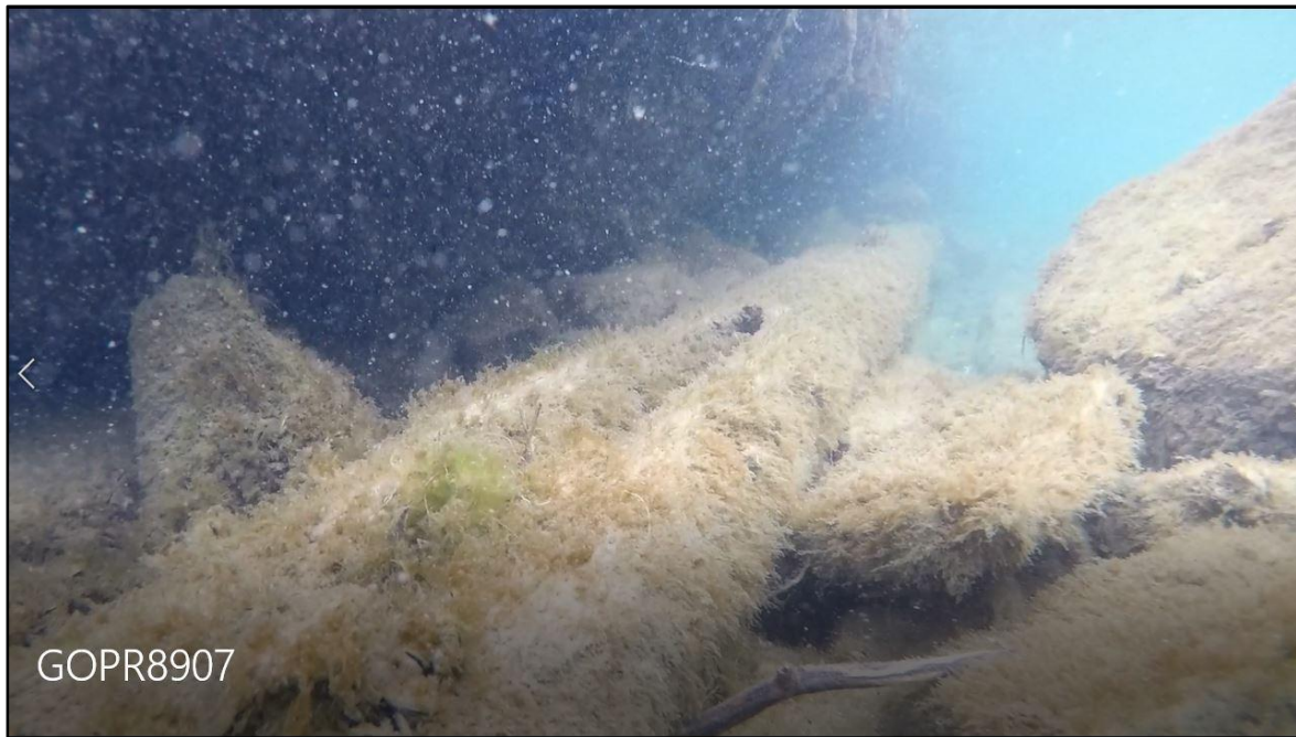
Photo 13: Failed timber cribbing SE shoreline parapet
