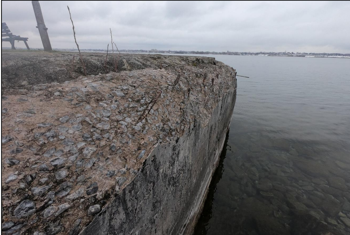
Photo 7: Existing concrete parapet, SW face
