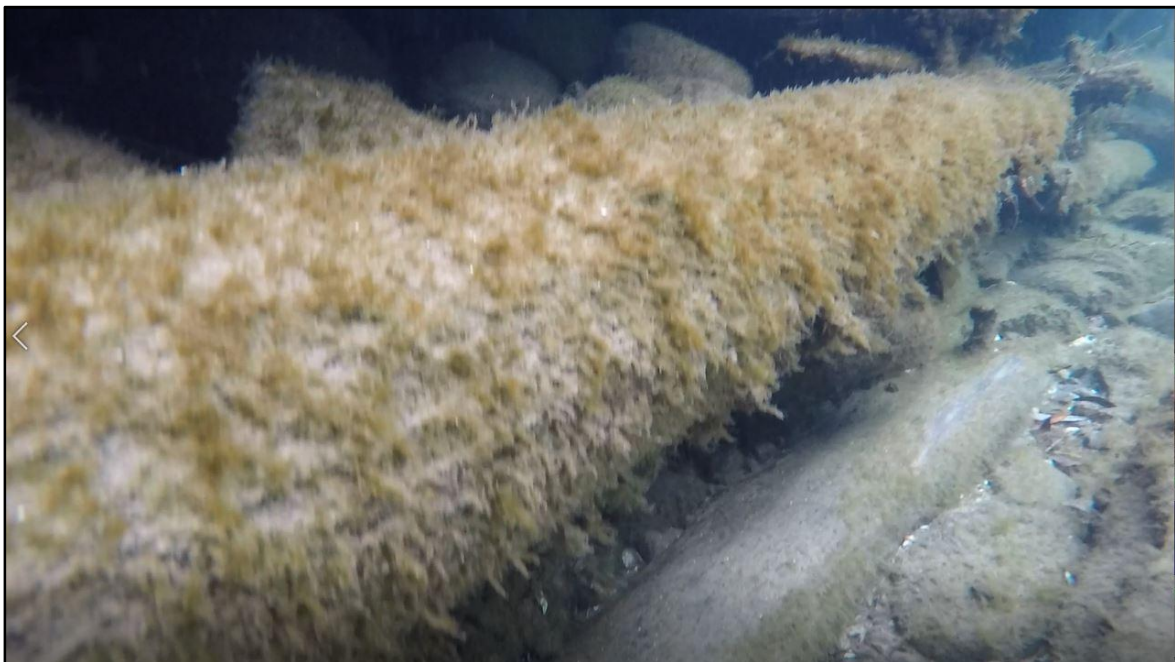
Photo 14: Partially failed cribbing SE shoreline parapet, stone fill behind
