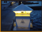
Protected KWH Counter
