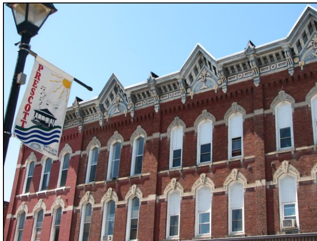
~ an architectural gem at King and Centre Streets ~
