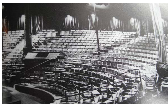
The Grand Chapiteau is 19 meters high, 51 meters in diameter. It is held up by four masts, each 25 meters tall and seats more than 2,500 people; the tent can require anywhere from 80–120 people to raise.
