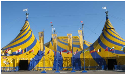
The Grand Chapiteau is 19 meters high, 51 meters in diameter. It is held up by four masts, each 25 meters tall and seats more than 2,500 people; the tent can require anywhere from 80–120 people to raise.
